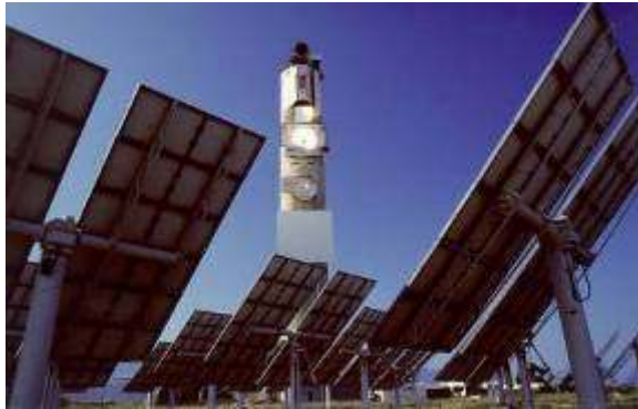
Solar thermal power plants
